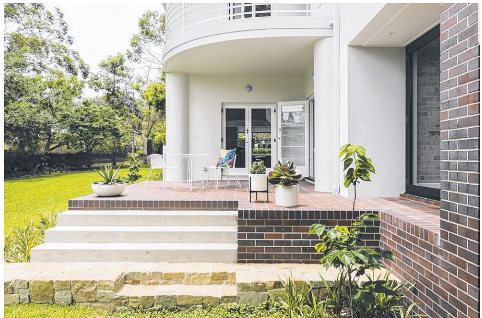
The original staircase and balustrade were restored.
